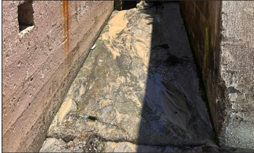
Photo 5: Typical Landing Erosion
