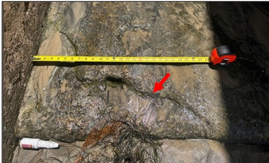
Photo 6: Additional Erosion at West End of Landing
