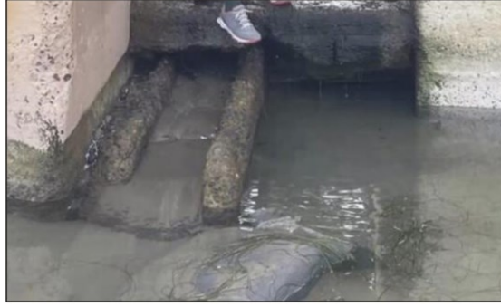
FIGURE 5: EXAMPLE OF SEASONAL SCOUR AT EXISTING WALKWAY BOTTOM LANDING
