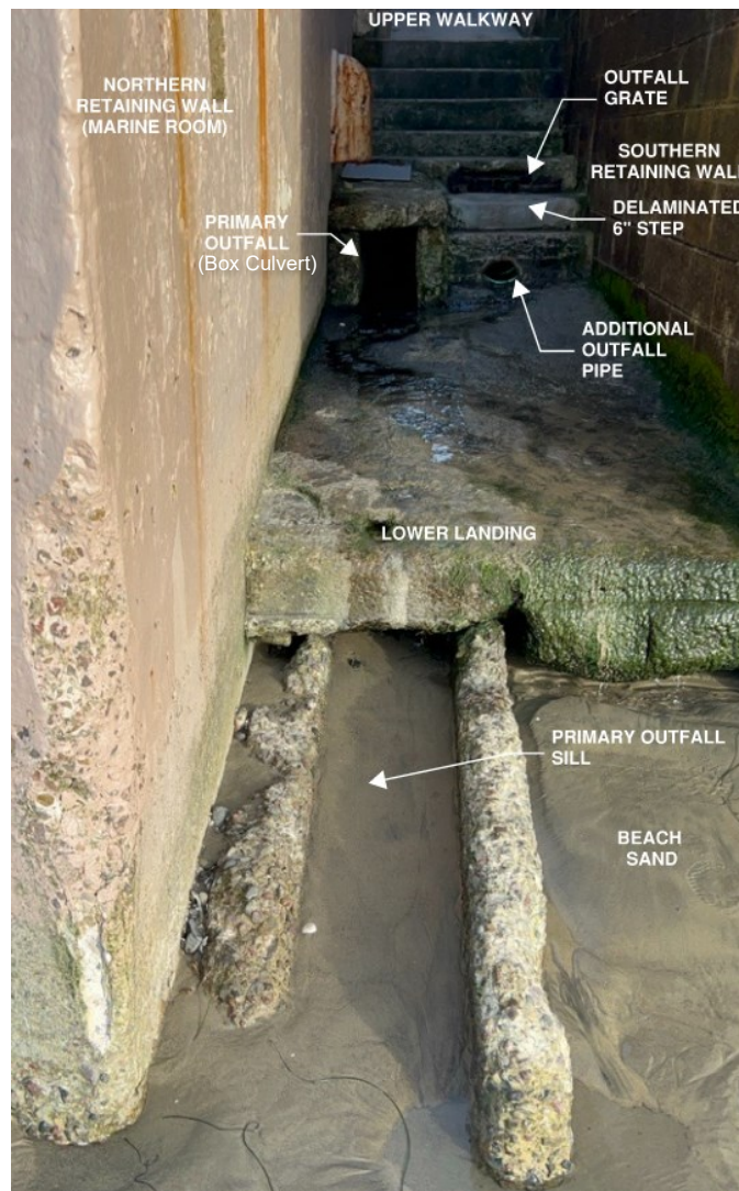
FIGURE 2: EXISTING WALKWAY PHOTO WITH KEY FEATURES IDENTIFIED
