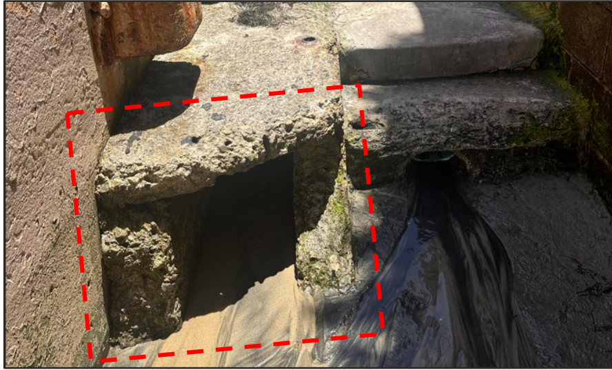
Photo 7: Box Culvert
