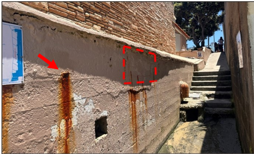
Photo 10: Closed Corrosion Spalls along the Northeast Retaining Wall
