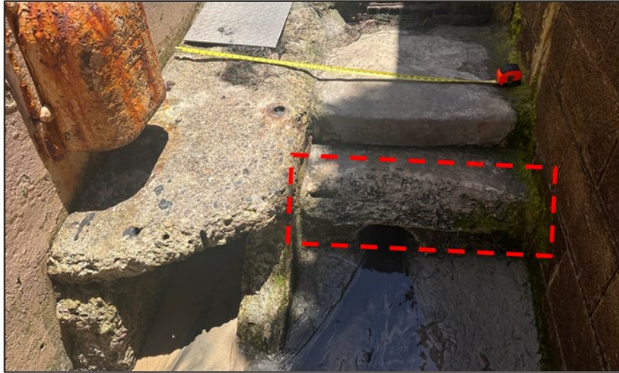
Photo 3: Erosion of Step 7
